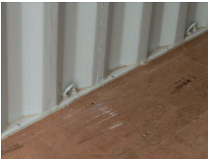
Container lashing points
